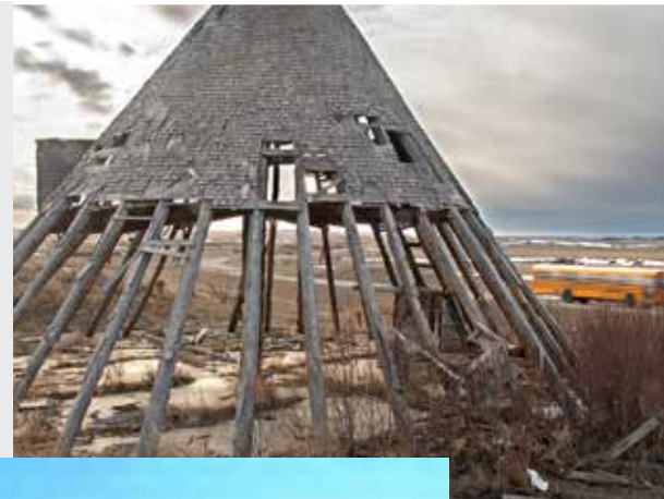
Busby tipi 2025; Today the structure has lost most of its shingles, leaving the wood exposed.
